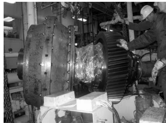
Photo 2 Installation of Pinion Shaft with Clutch
