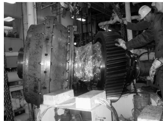
Photo 2 Installation of Pinion Shaft with Clutch
