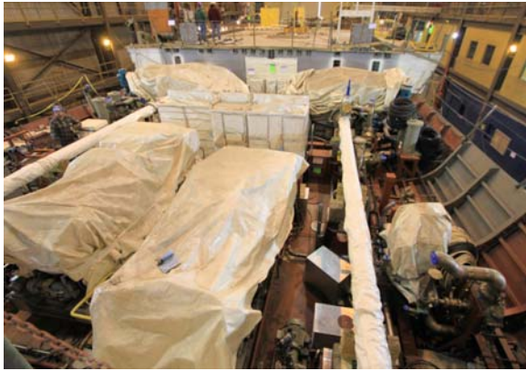
Photo 1 LCS 3 MPDEs and Gear Coupling Shafts to Splitter Gearboxes (Looking Aft)
