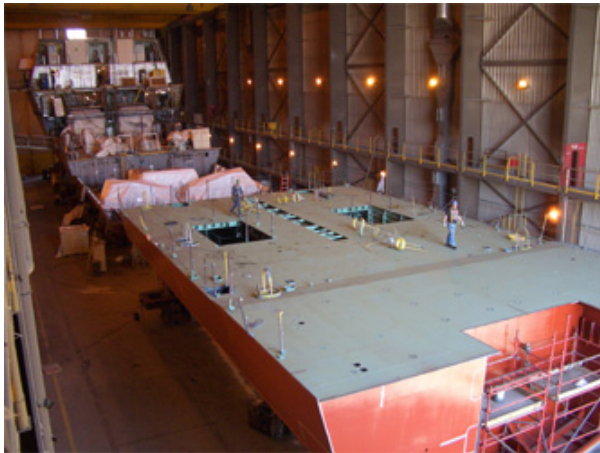
Photo 5 Hull Under Construction
