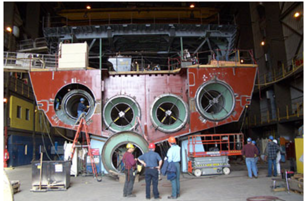
Photo 7 Preparation for Waterjet Installation
