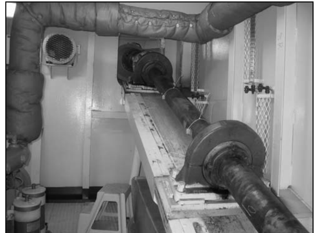
Photo 3 Aft Two Bearings on Lineshaft
