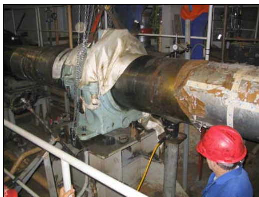
Figure 2 Jack-Up Load Test on Lineshaft Bearing
